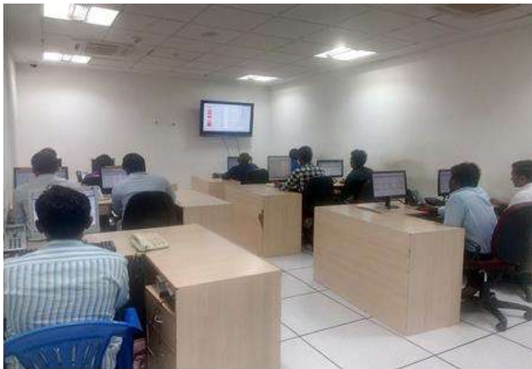
TNSWAN Network Operations Centre
