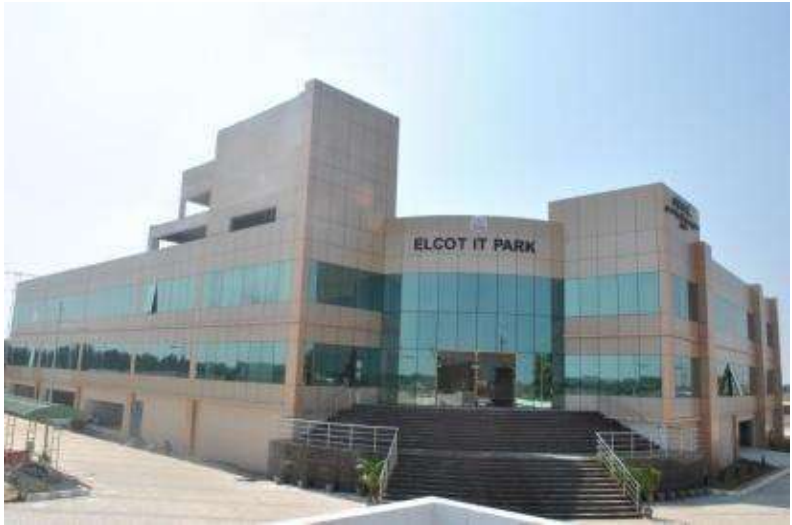
ELCOT IT Building, Navalpattu,Trichy
